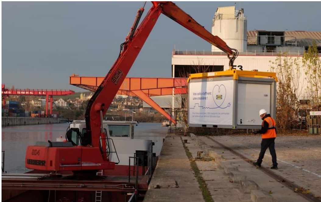
Fig 3.5: The Swedish company Ikea uses the Fludis transport services to connect its depot situated at the Port of Gennevilliers, and the Paris centre where it has many customers.
