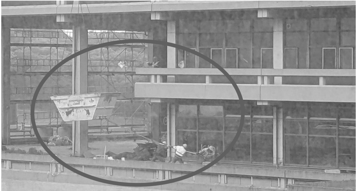
Figure 3.1: Throwing debris into a container, above of other workers (Picture by Felix Thewes, 2022)
