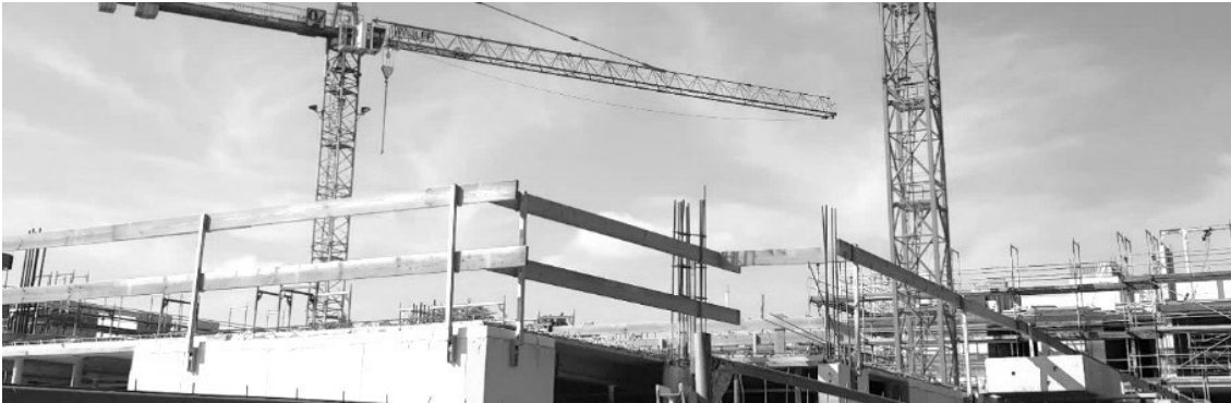
Figure 3.3: Fall Protection (red planks) to prevent falls from heights
