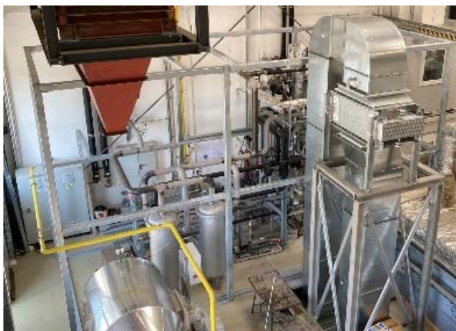
Figure 14: fire-resistant enclosure steelframe as built.
