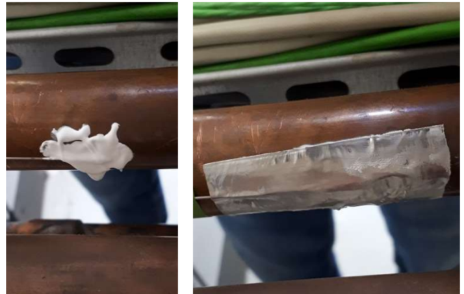
Figure 3: Installation of Ø 0.75 mm thermocouple at the surface of the pipe with a layer of thermal paste (right) and covered with aluminium tape (left).
