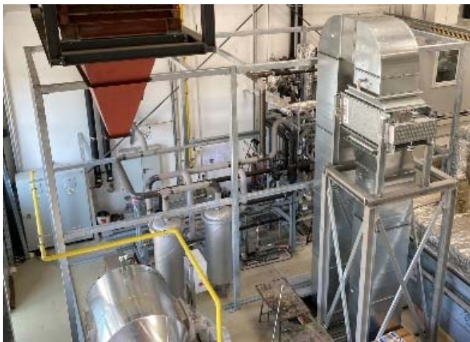
Figure 14: fire-resistant enclosure steelframe as built.
