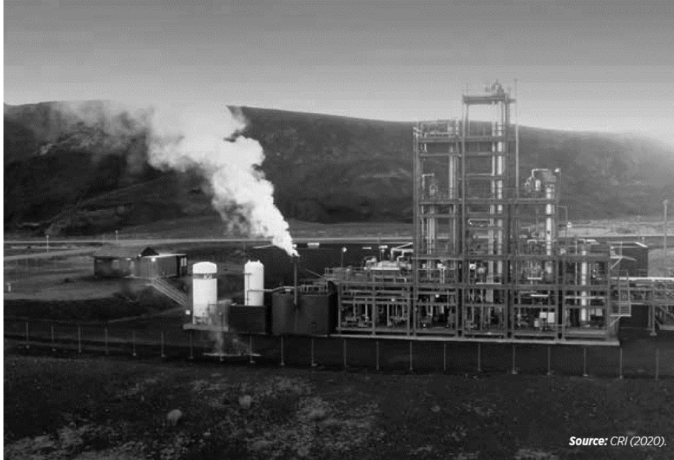
Figure 2-11: 4,000 t/year Methanol Production of CRI in Iceland (see also Chapter 2.3.1)
