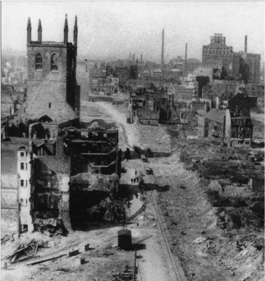
Figure 3: Kampstraße in Dortmund, with the destroyed Petrikirche, in the background the Union Brewery, photo: Dortmund municipal archives
