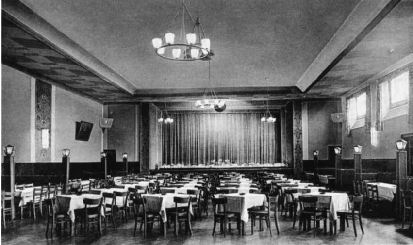
Figure 11: Hall of the “Postkutsche” in Dortmund-Aplerbeck, photo: private collection
