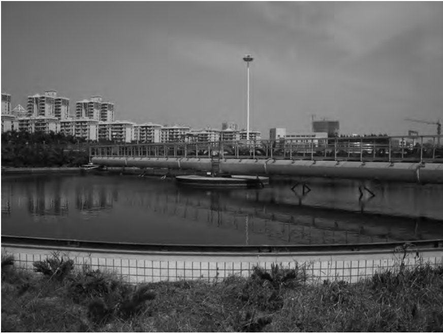
(1) Modern sewage treatment plant, Xiamen/Fujian province.
