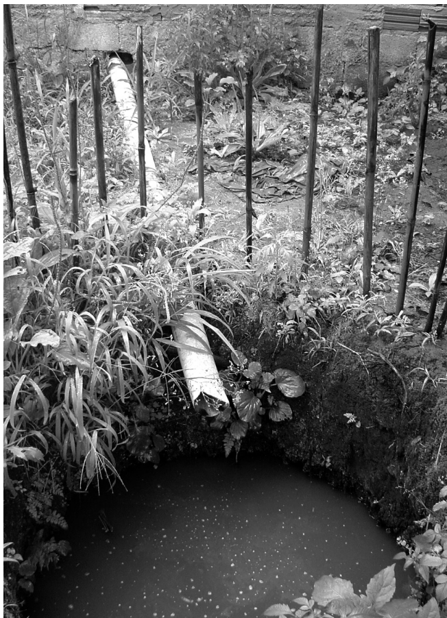
(2) Cesspit used for wastewater disposal in a poor community situated at the southern region of Parelheiros District (Municipality of São Paulo). It is not unusual to find cesspits dug up to the water table, bringing pollution to groundwater that will be exploited by nearby dug wells.
