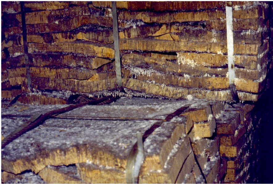
Figure 1-5 Mildewed cork planks due to inadequate drying conditions after boiling (photo: Rudolf Ohlinger GmbH)
